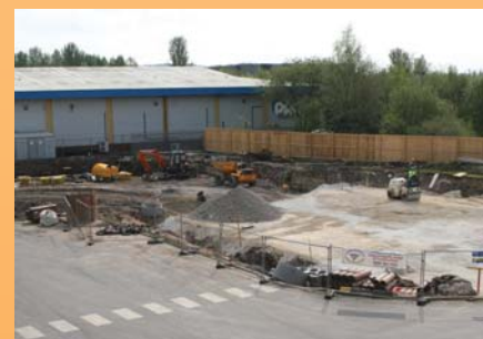
Work on the warehouse gets under way
